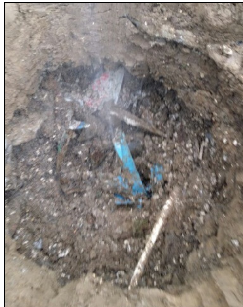
Moled solution – launch and reception pits
